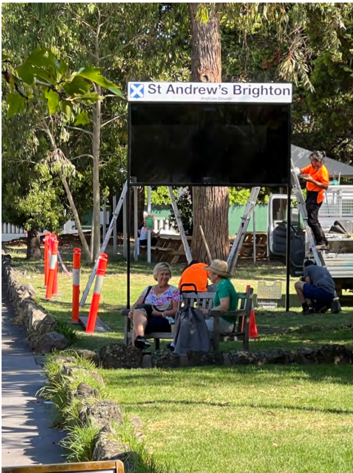
New sign installation
